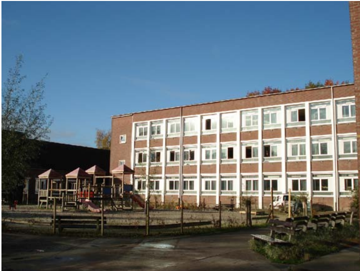
Sint Truiden Reception Centre. Accomodation
