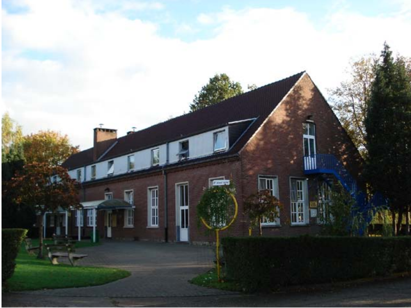
Sint Truiden Reception Centre. Restaurant
