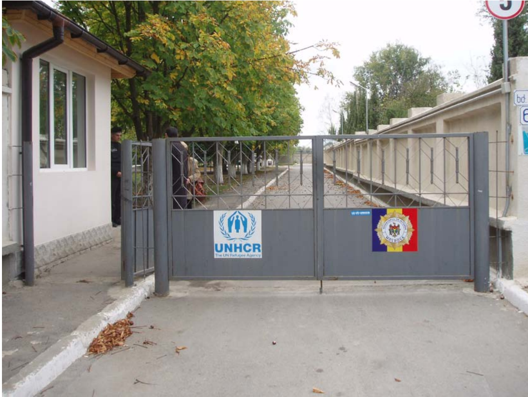
Entrance at the Reception Center.
